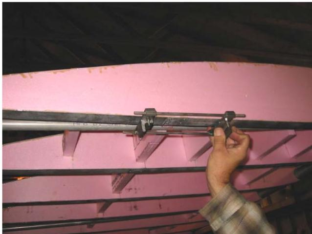
Homemade stretcher tool to place the aluminum bands. (DJ)
